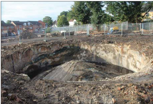
Plate 3. Remediation, interior base of gas holder.
