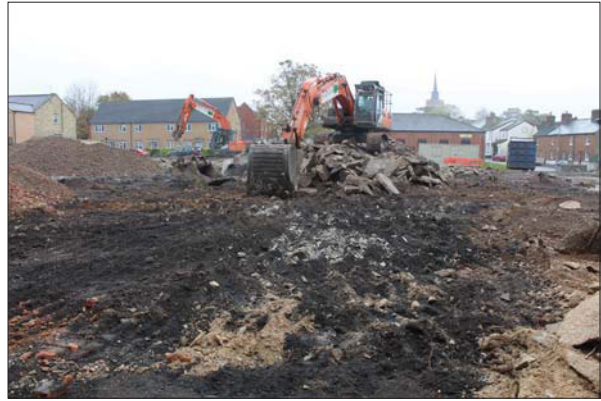
Plate 1. Remediation, working progress.
