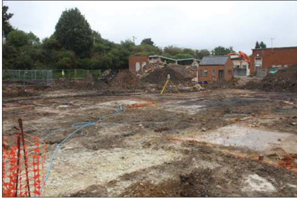
Plate 1. Remediation, excavated level under concrete slab
