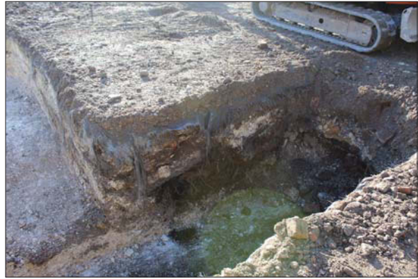
Plate 6. Groundworks, variety of modern fill exposed in section during groundworks.
