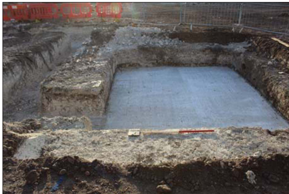
Plate 7. Groundworks, concreted lift base of E building, Scale: 1m.
