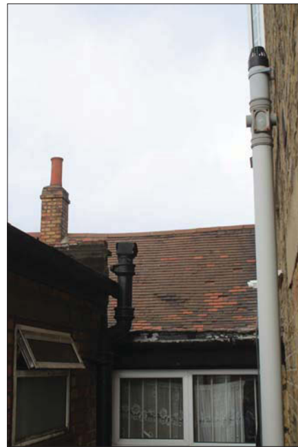
Plate 2. Pitched roof detail, looking north-west.
