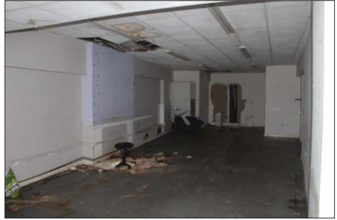
Plate 18. Room 2, general view, looking south-east.
