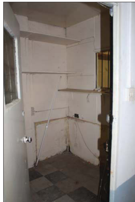
Plate 28. Room 5, inserted store room, looking north-west.
