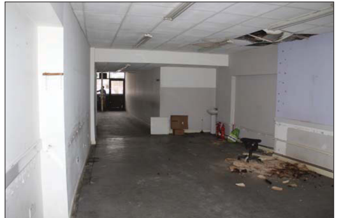
Plate 12. Room 2, general view to front, looking north-east.
