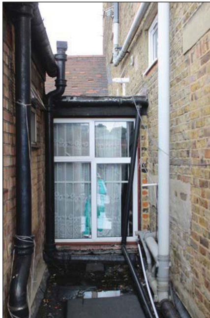
Plate 11. Window detail, looking north-west.
