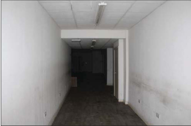
Plate 5. Room 2, general view, looking south-east.
