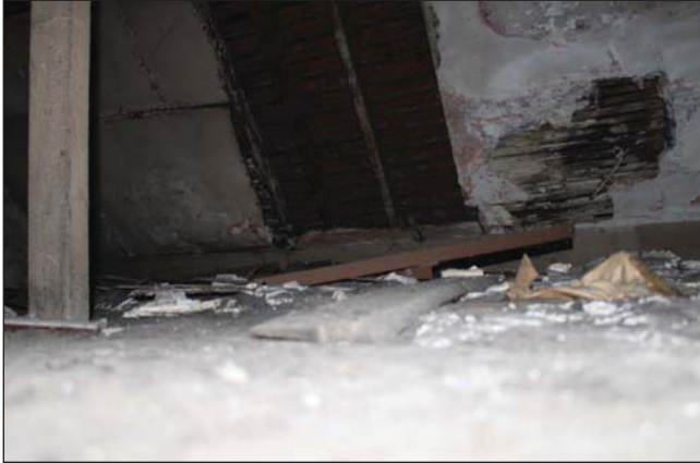
Plate 9. Attic, roof detail, looking north-west.
