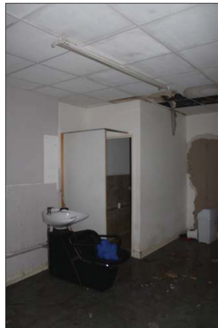
Plate 24. Room 2, inserted toilet, looking south-east.
