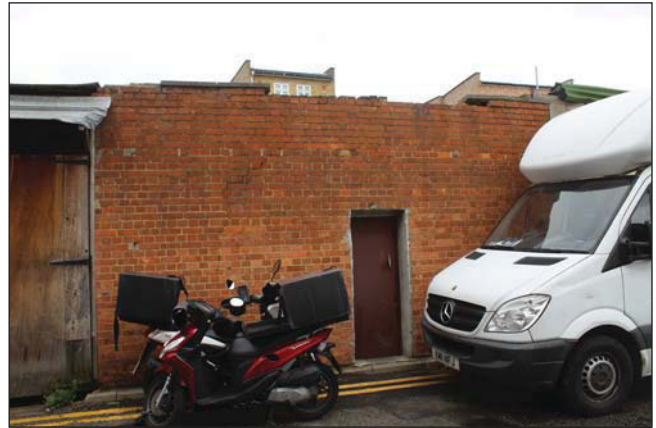
Plate 30. Rear entrance of 104, looking northe-ast.
