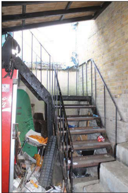
Plate 29. Room 6, stairs to first floor, looking south-east.
