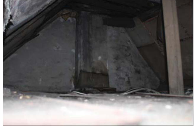
Plate 10. Attic, gable end and chimney stack, looking north-west.
