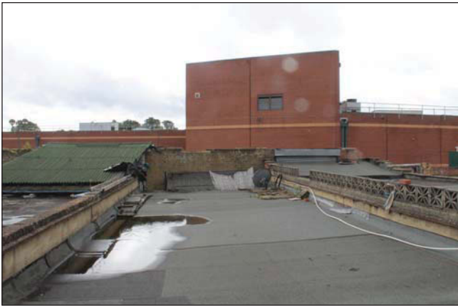
Plate 31. view across flat roof to stairs, looking south-east.
