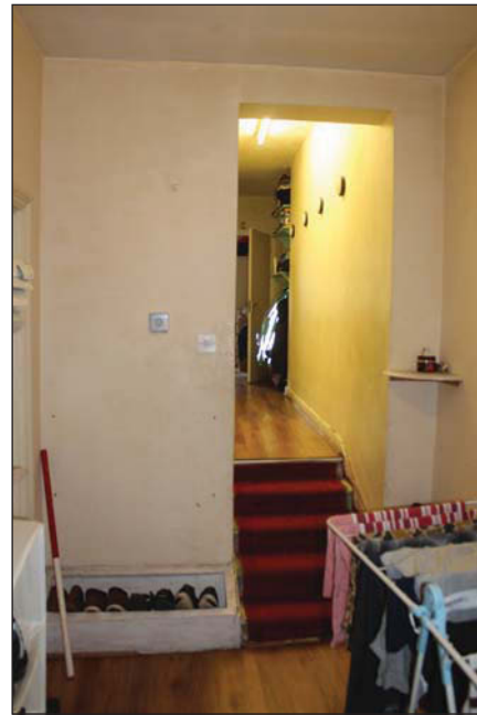
Plate 14. Room 8, stair detail, looking south-east.
