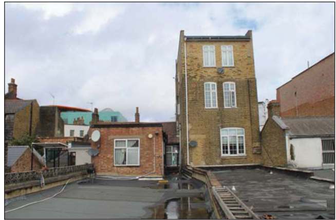
Plate 32. view across flat roof to rear of building, looking north-west.
