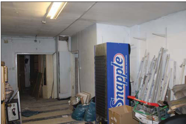
Plate 27. Room 5, general view showing inserted room, looking north-east.
