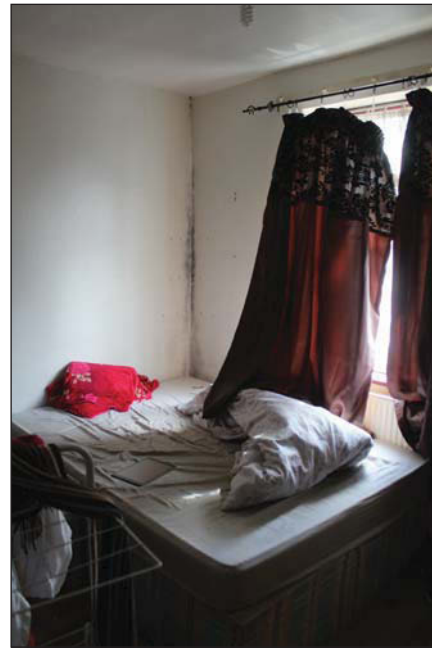
Plate 22. Room 13, general view, looking south-west.
