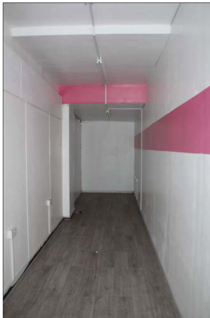
Plate 3. Room 1, general view, looking south-east.
