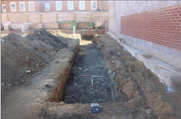
Plate 1. Foul water service trench, looking East, Scales: 1m.
