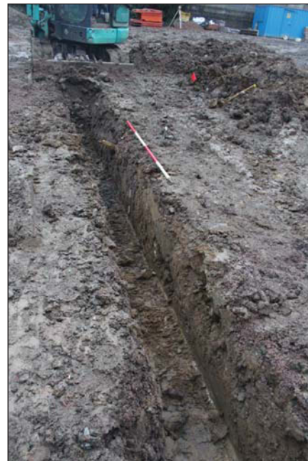
Plate 4. Utility trench, looking South, Scale: 2m.
