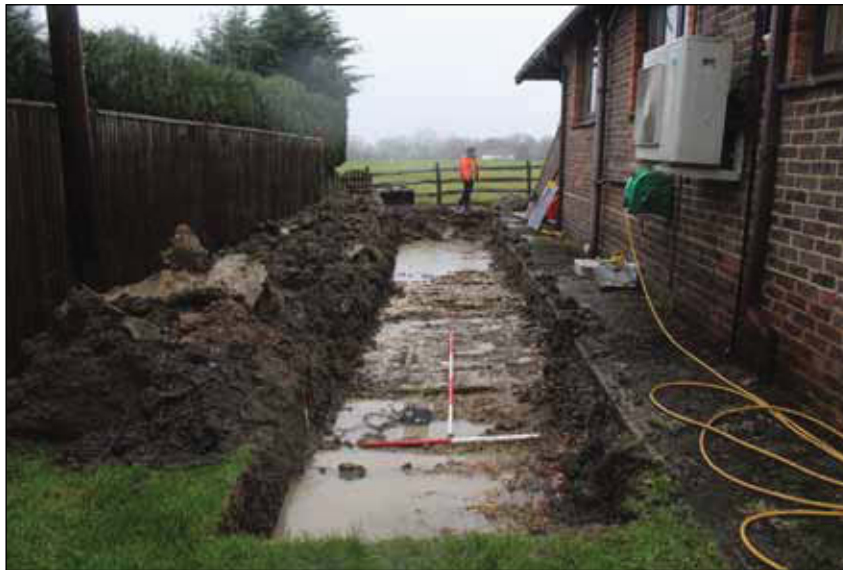
Plate 1. Trench 1, looking East, Scales: 2m, 1m and 0.30m.
