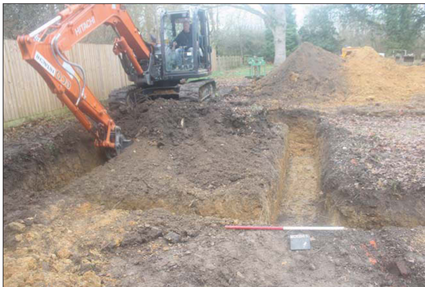
Plate 2. Excavated footing in progress on garage, looking North West, Scale: 1m.
