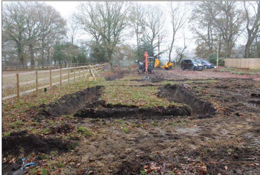
Plate 1. View over excavated footings, looking South East.
