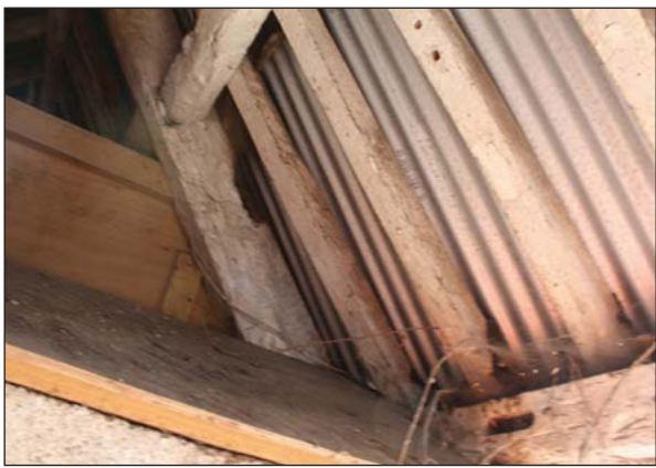
Plate 39. Interior roof of lean-to showing wooden beams. Looking East.
