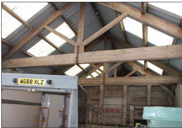
Plate 81. Frame of roof supporting corrugated steel looking south. Looking South.
