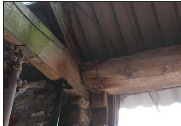
Plate 84. Close up of wooden beam and roof supporting structure. Looking East.
