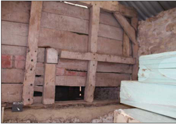
Plate 79. Close up of western corner of main barn. Looking West.
