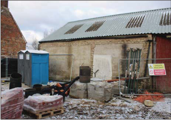
Plate 1. View of outer south eastern elevation with rendering. Looking West
