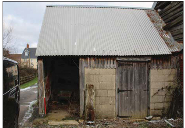
Plate 16. View of lean-to south eastern elevation, two wooden doors on and steel roof. Looking North West, Scales: 1m
