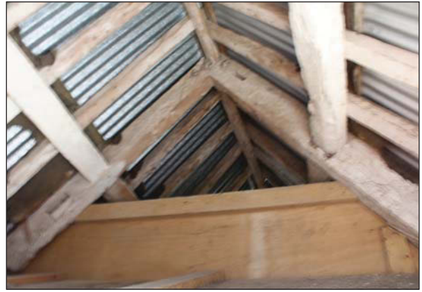
Plate 38. Interior roof of lean-to showing wooden beams. Looking North East.
