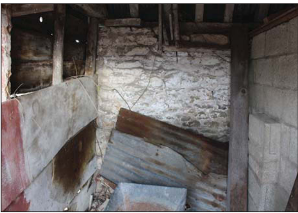
Plate 33. Interior of north western wall of lean-to. Looking North West.
