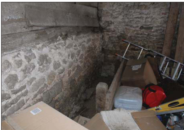
Plate 47. Interior of south eastern chamber of barn. Looking South East.
