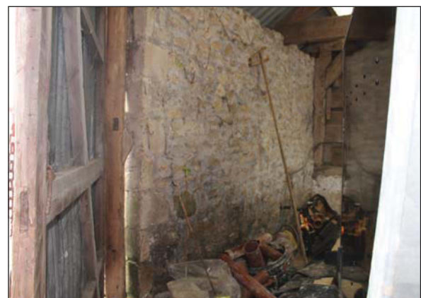
Plate 82. South corner of main barn. Looking South.
