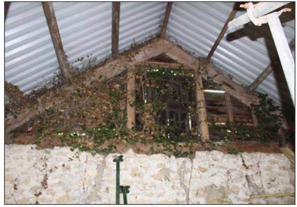
Plate 62. Close up of hay loft hatch. Looking North East.
