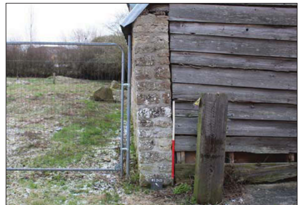
Plate 30. Sidelong view of north western elevation. Looking North East. Scale: 1m
