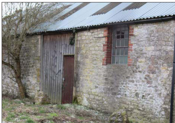
Plate 23. Close up of north western barn doorway and large window. Looking East.
