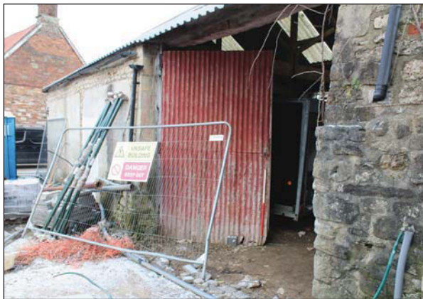
Plate 9. South Eastern doorway, corrugated steel door. Looking West. Scale: 1m
