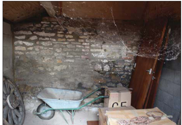
Plate 42. Interior of north west wall of lean-to. Looking North West.
