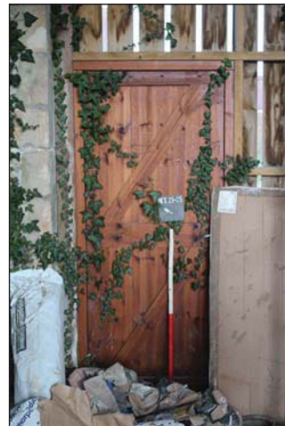
Plate 72. Close up of north western door. Looking North West. Scale: 1m
