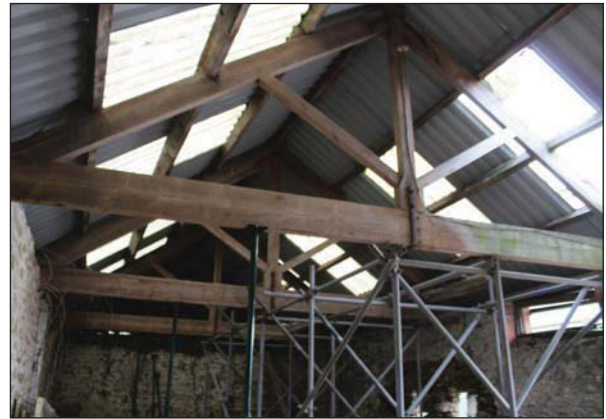
Plate 58. Interior main barn roof structure. Looking South East.
