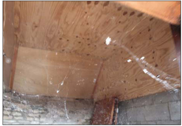
Plate 44. Ceiling of lean-to room showing modern ply board. Looking North.
