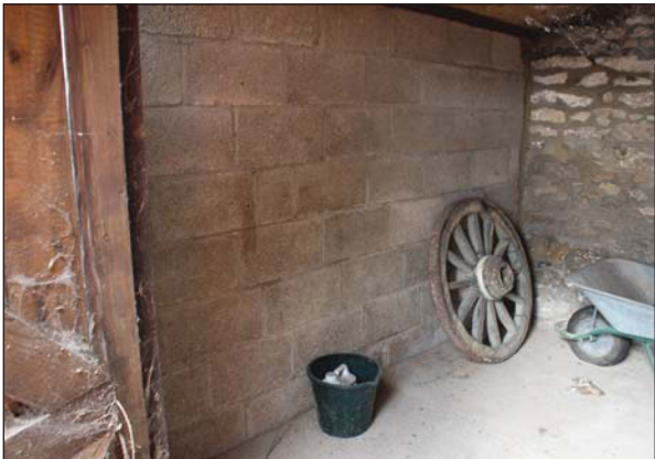
Plate 41. View of interior breeze block dividing wall. Looking West.
