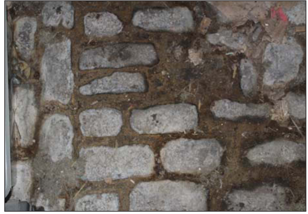
Plate 50. Cobbled floor of western barn chamber.
