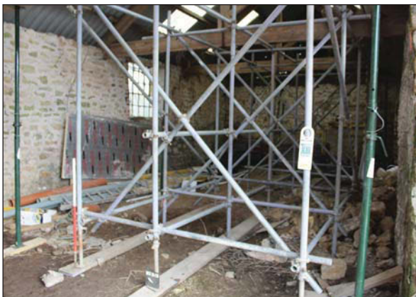
Plate 59. Interior of main barn, facing northern corner. Looking North. Scale: 1m
