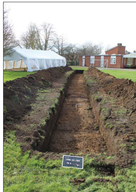
Plate 4. Trench 5, looking South West Scales: 1m
