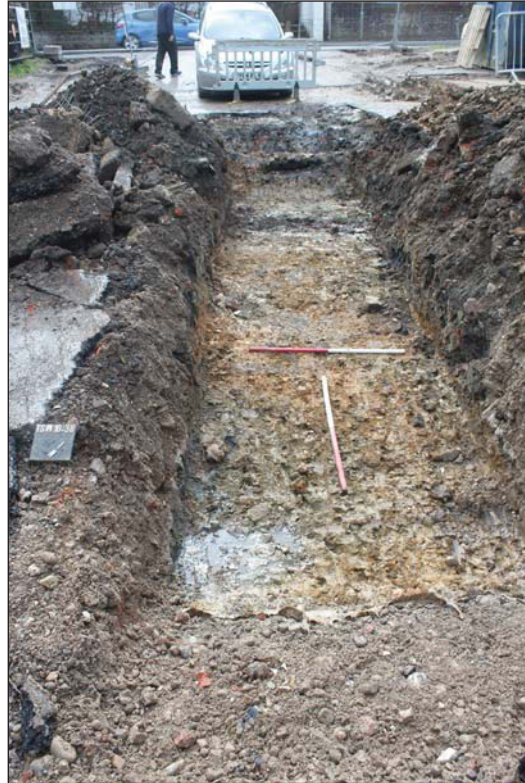
Plate 4. Trench observed in watching brief area, looking north-west, Scales: 2x1m.
