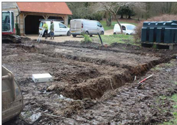
Plate 1. Progress of footing, looking South East, Scale: 1m.
