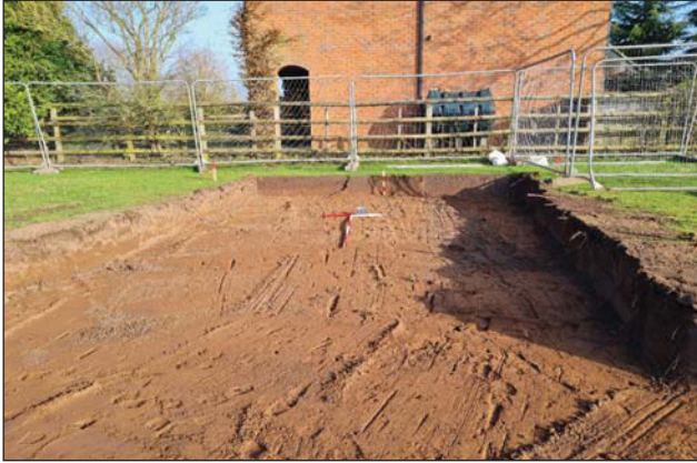
Plate 1. Turning bay and section, looking east, Scales: 2m, 1m and 0.5m.
