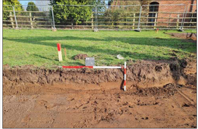
Plate 2. Access road (north), looking east, Scales: 1m and 0.5m.
