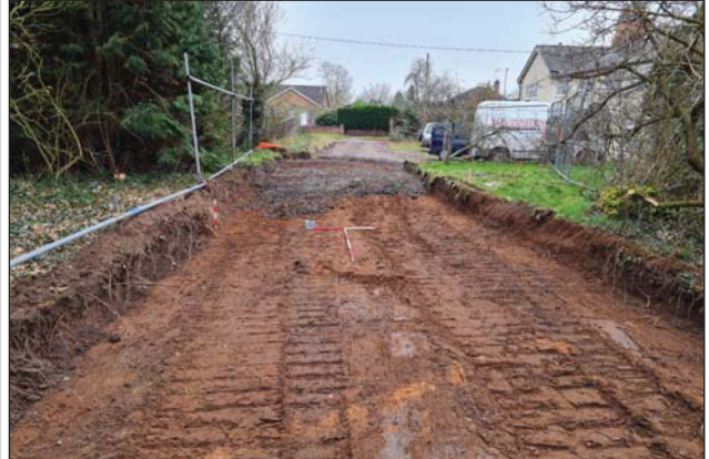
Plate 2. Access road (southern end), looking south, Scales: 2m and 1m.
