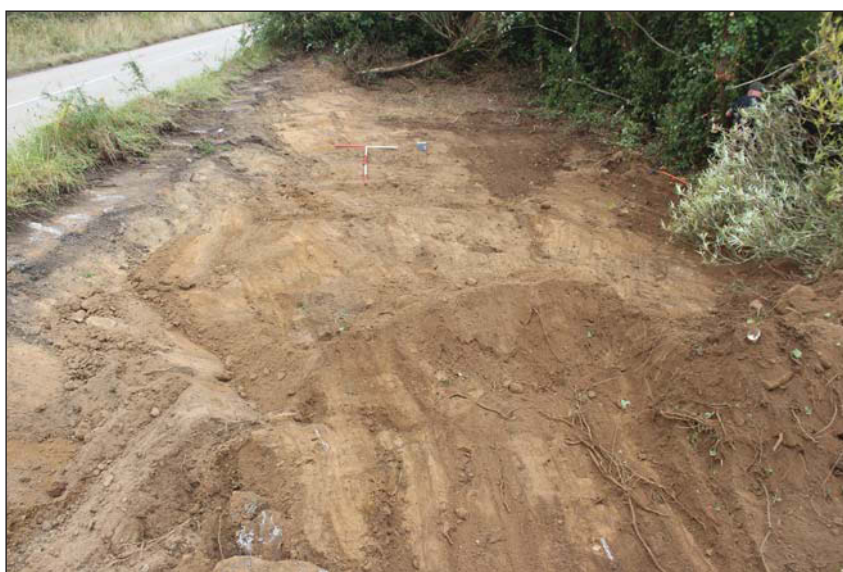
Plate 4. Shot of ground reduction area, looking north. Scales: 2m and 1m.
