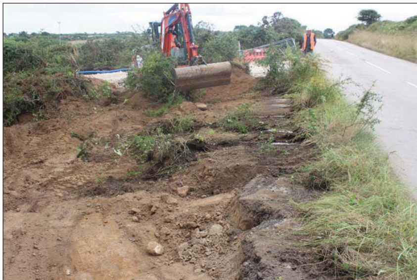
Plate 3. Working shot of ground reduction area, looking south.
