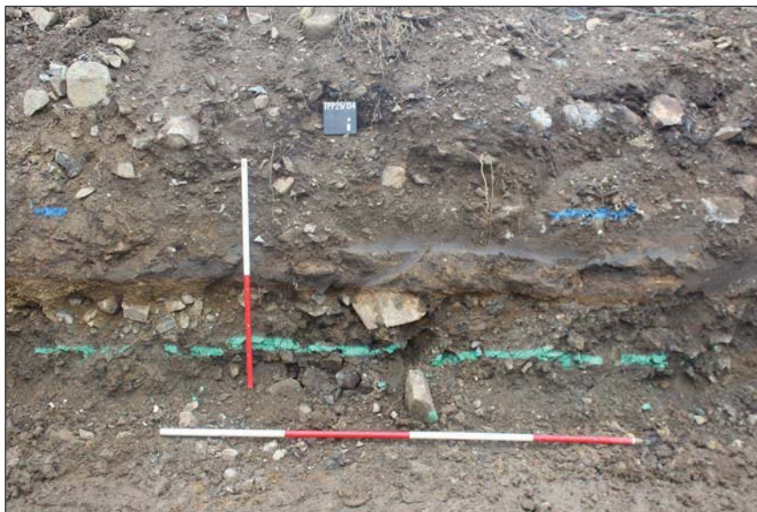
Plate 2. Section of access road, looking south. Scales: 2m and 1m.
