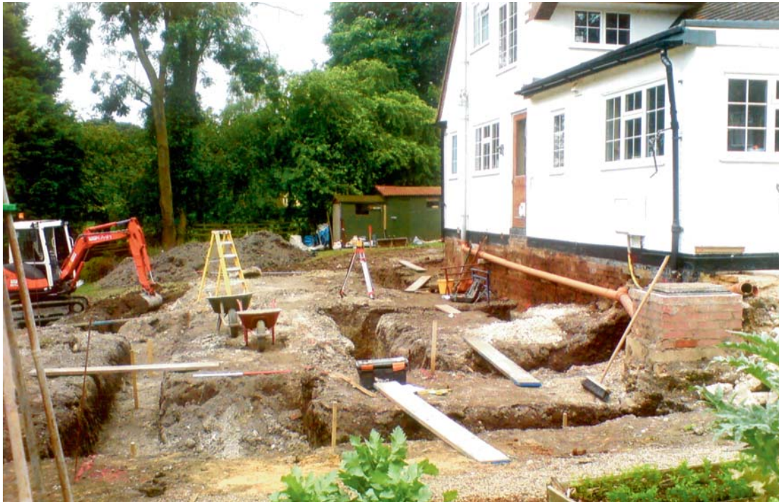
Plate 1. General rear footings for extension and patio, looking south.
