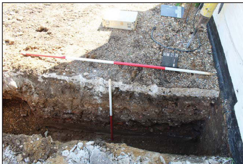
Plate 2. Representative section of footing trenches, looking south, Scales: 2m and 1m.
