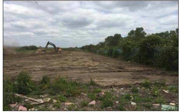
Plate 8. Southern part of new training pitches area, looking East, showing trackway 53.
