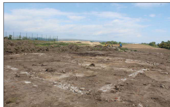
Plate 10. Building 55, looking North-east.
