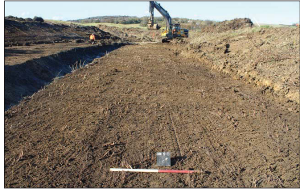
Plate 2. Haul road crossing point 2, looking North-west. Scale: 1m.
