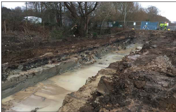
Plate 3. General view of northern culvert, looking North-east towards site entrance.
