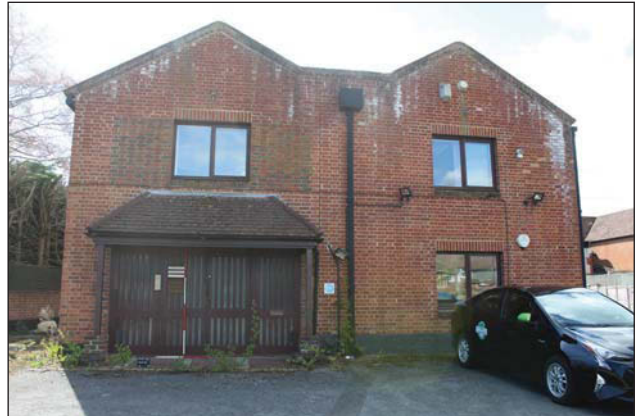
Plate 10. Office block north elevation, looking S, Scales: 1m and 2m
