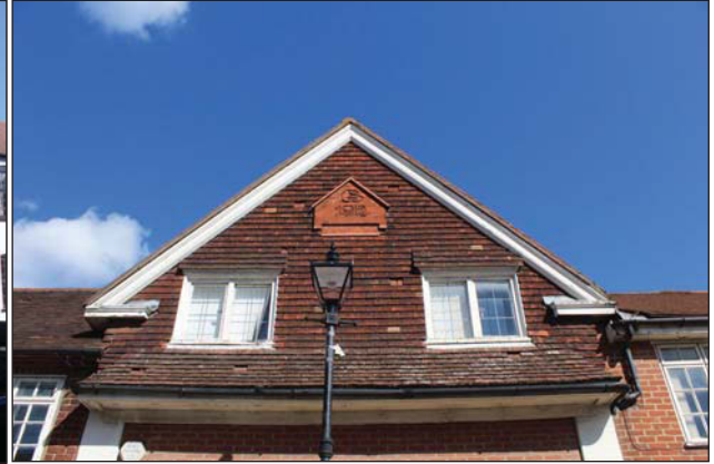
Plate 2. Front elevation, central gable, looking NW.
