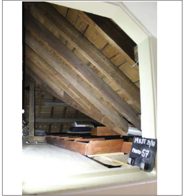
Plate 22. Roof space, looking S, Scales: 1m and 2m.
