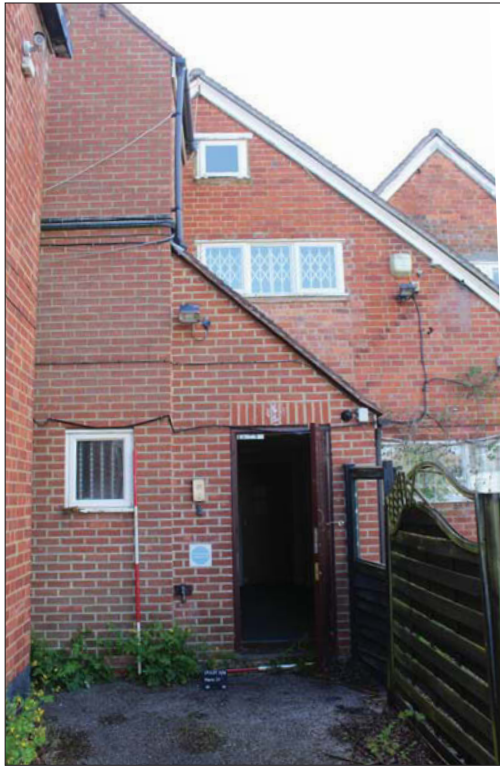
Plate 9. Rear of number 19, looking SE, Scales: 1m and 2m.
