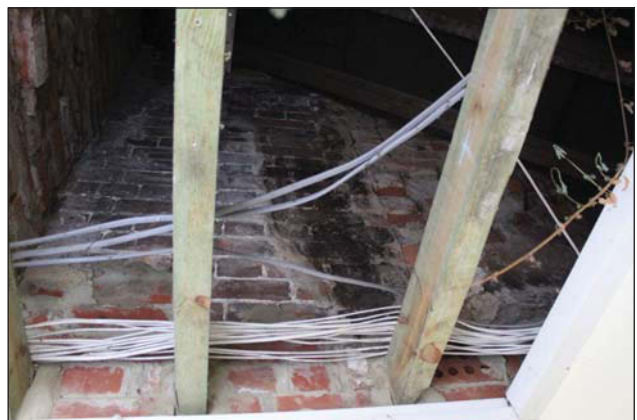
Plate 12. Ceiling room 2, looking SE.
