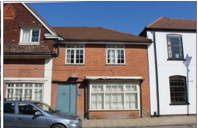
Plate 4. Front elevation, looking NW
