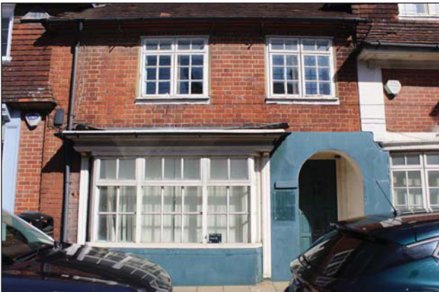
Plate 3. Front elevation, looking NW.
