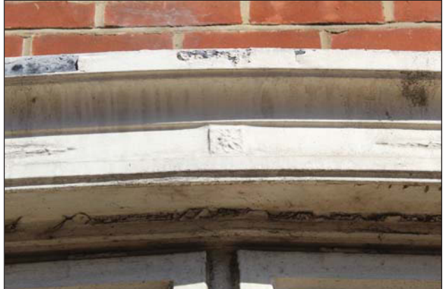
Plate 6. Front elevation, detail of bay window (centre), Looking NW.
