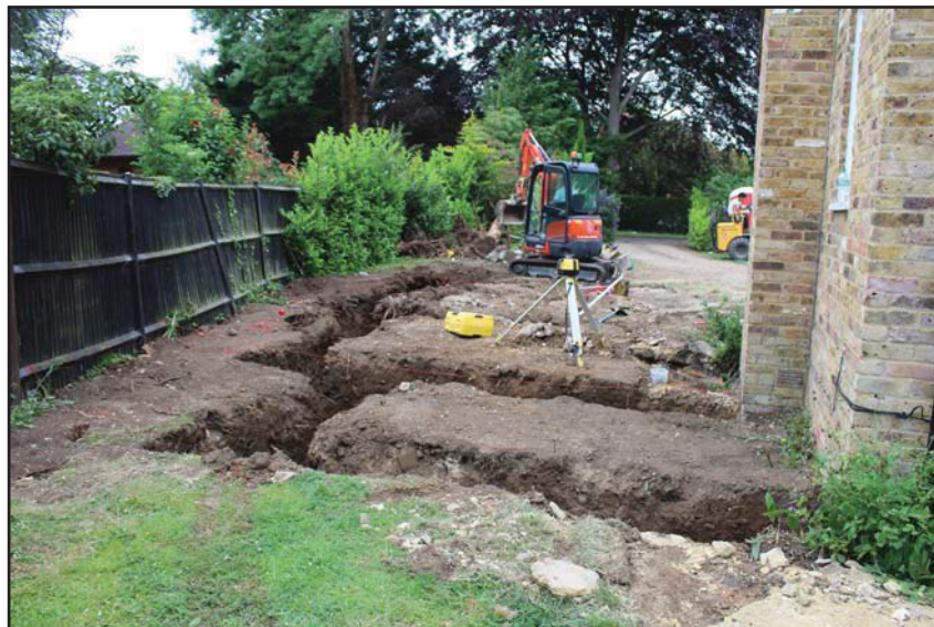
Plate 1. Foundation trenches under excavation, looking west.
