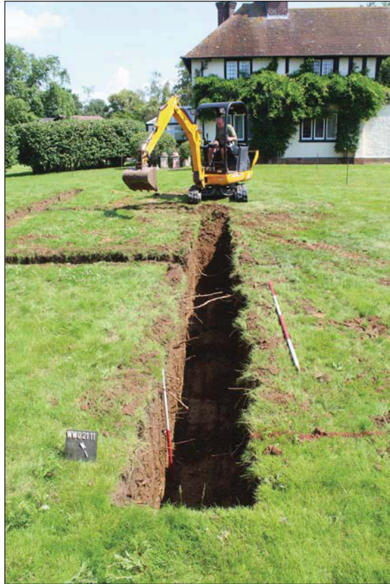
Plate 1. Foundation Trench , looking North, Scales: 2m and 1m.
