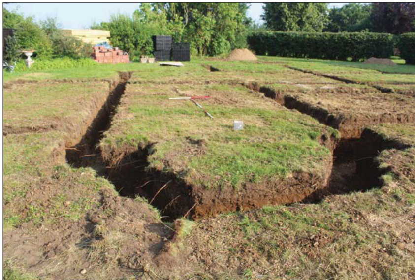
Plate 2. Foundation Trenches, looking North West, Scales: 2m and 1m.
