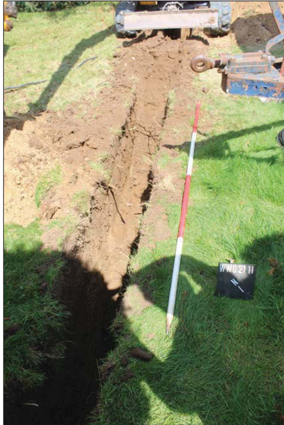
Plate 3. Drainage Trench, looking North East, Scales: 2m.
