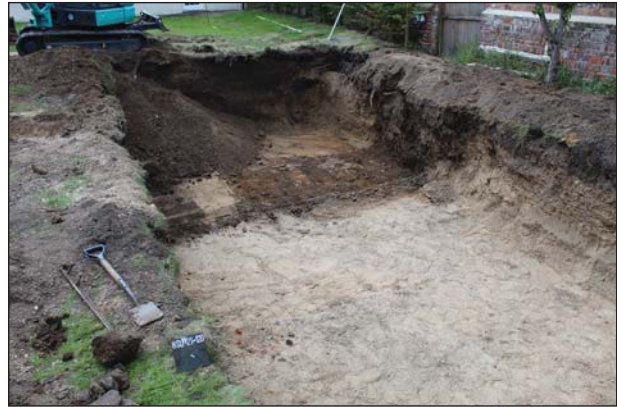
Plate 2. Excavation in progress, looking North West.
