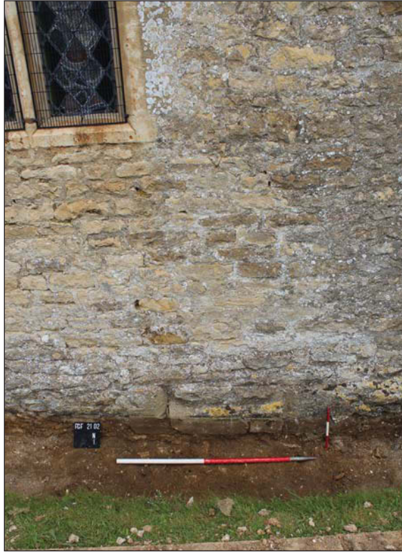
Plate 1. South circuit drain, Reconstructed wall above older foundation of chancel, looking North, Scales: horizontal 2m, vertical 0.3m.
