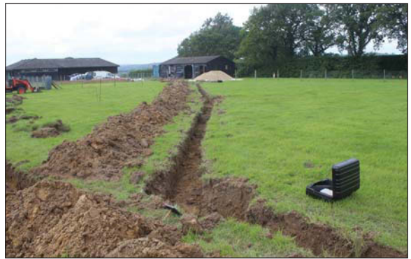
Plate 4. General view of foul service trench, looking North-west.
