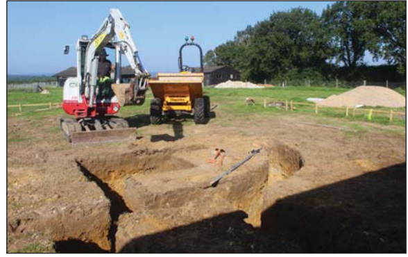
Plate 2. General view of house footings, looking North-west.
