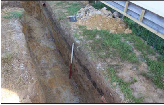
Plate 1. Easternmost house footing trench, looking East. Scale: 1m.
