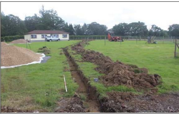
Plate 3. General view of foul service trench, looking South-east.
