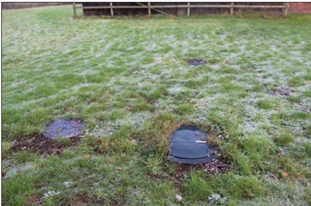
Plate 3. Man hole covers in southern part of survey area.
