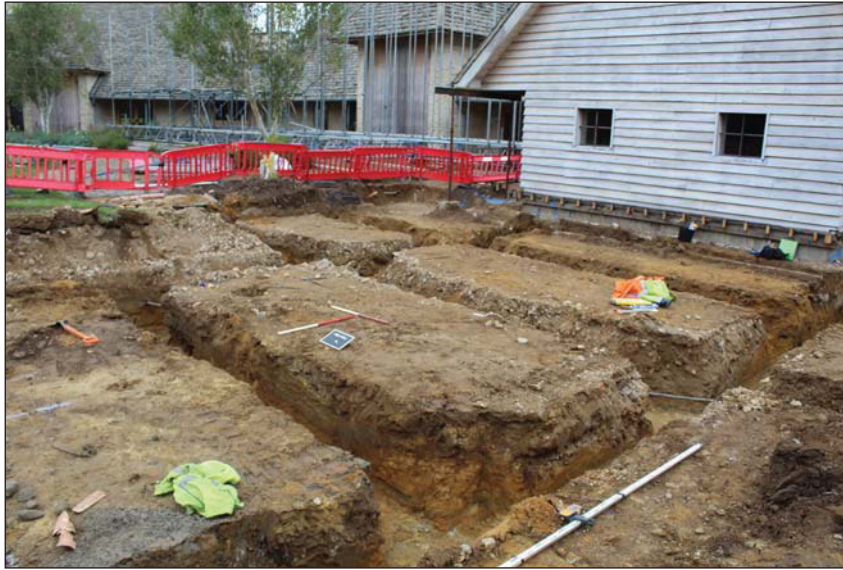
Plate 1. Extension footings, looking North West, Scales: 1m x2.
