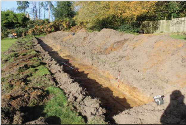
Plate 3. Trench 16, looking North West, Scales: 2m, 1m and 0.5m.
