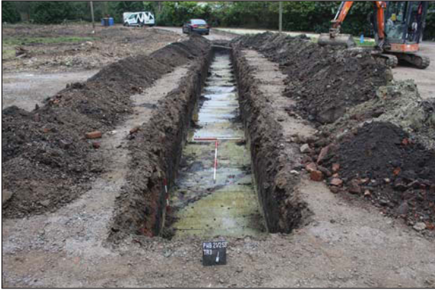
Plate 1. Trench 3, looking South South West, Scales: horizontal 2m and 1m, vertical 0.5m.
