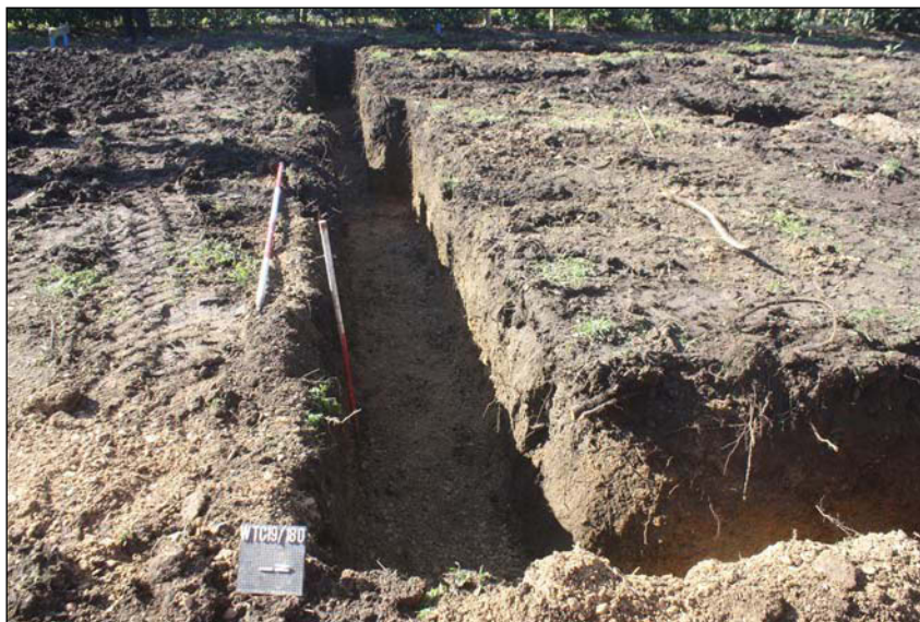
Plate 2. Southern trench footings, looking west, Scales: 2m and 1m.
