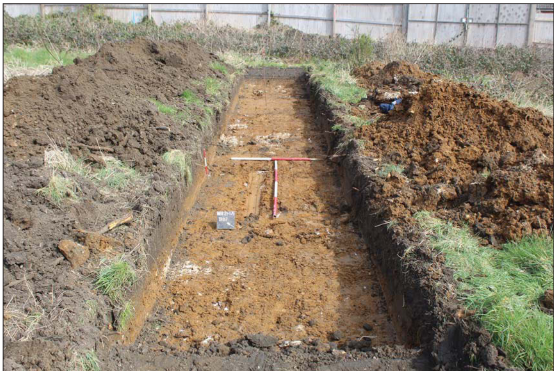
Plate 4. Trench 7, looking North East, Scales: horizontal 2m and 1m, vertical 0.3m.
