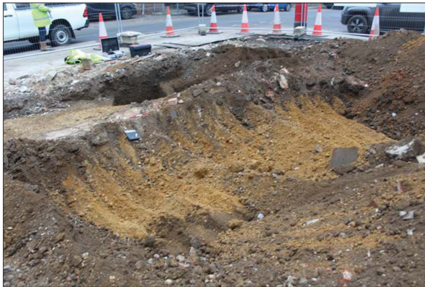
Plate 6. Remediation adjacent to existing footing,, looking North, Scale: 0.3m .
