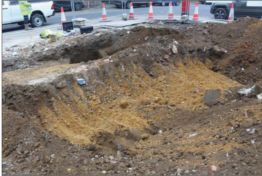
Plate 1. Ground strip adjacent to existing footing, looking North West, Scale: 0.3m.
