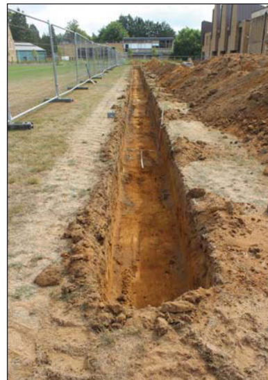
Plate 4. Service trench, looking E, Scales: horizontal 2m and 1m, vertical 1m.
