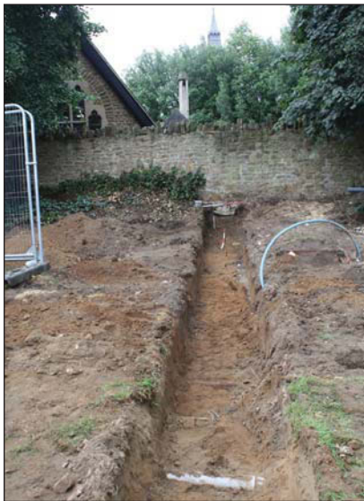
Plate 3. Service trench, looking S, Scales: 2m and 1m.
