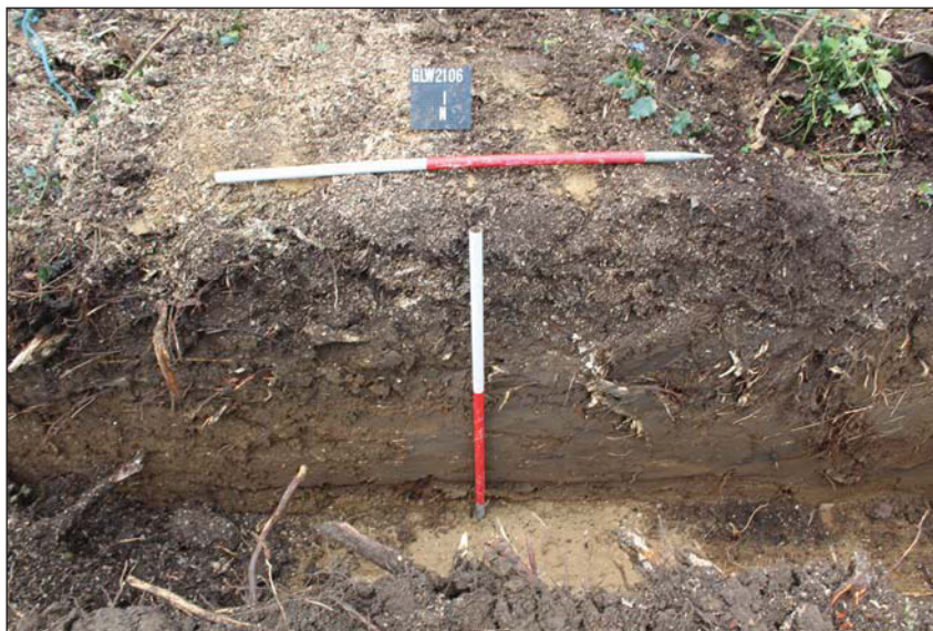
Plate 2. New garage footing, looking S, Scales: horizontal 1m, vertical 1m.
