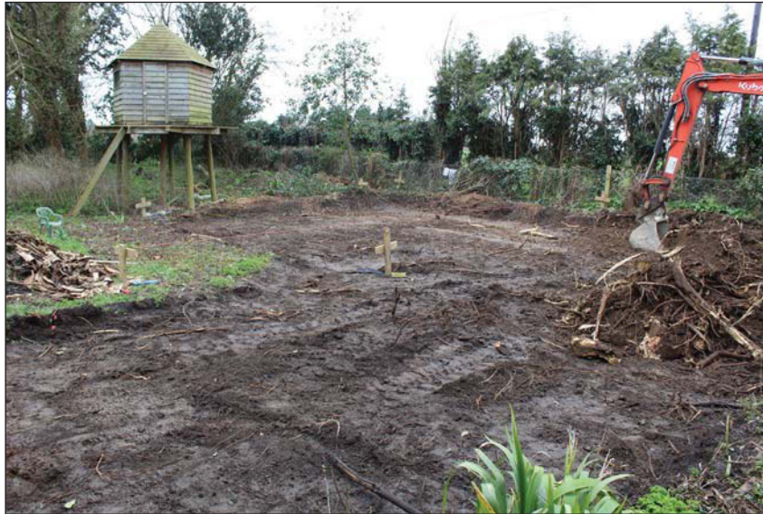
Plate 1. Area stripped viewed over location of garage, looking SW.
