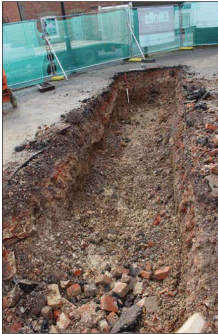
Plate 5. Trench dug through existing car park looking south west, Scales: 1m.
