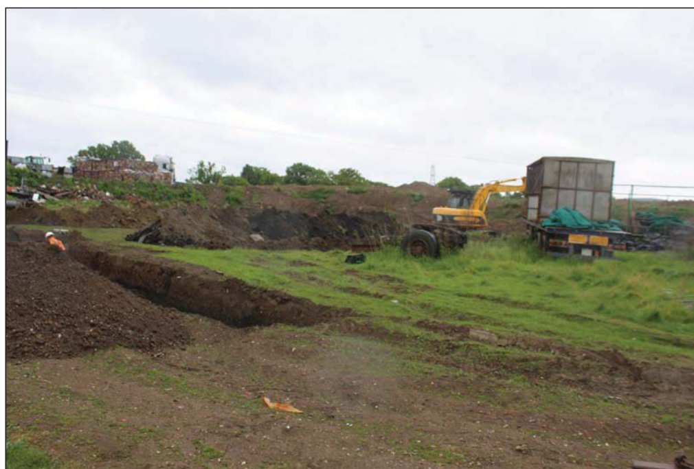
Plate 6. Trench 4, looking east..
