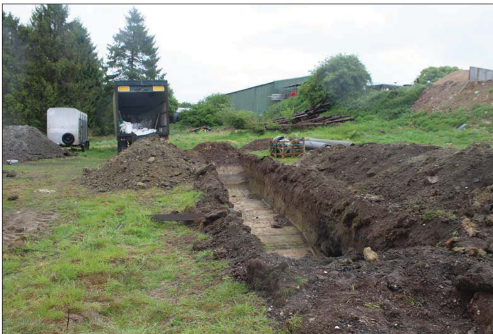
Plate 5. General view of site looking north
