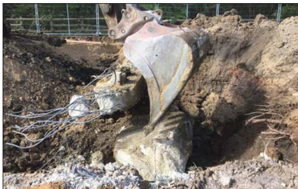
Plate 1. General shot showing the removal of a ground beam to expose the concrete pad beneath, looking South-west.
