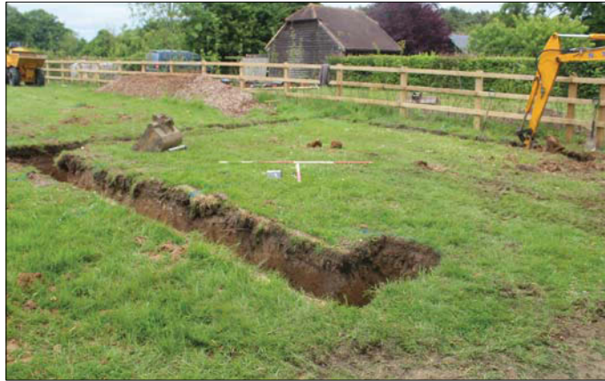
Plate 1. Location of new Garage excavation, Scales: 2m and 1m.
