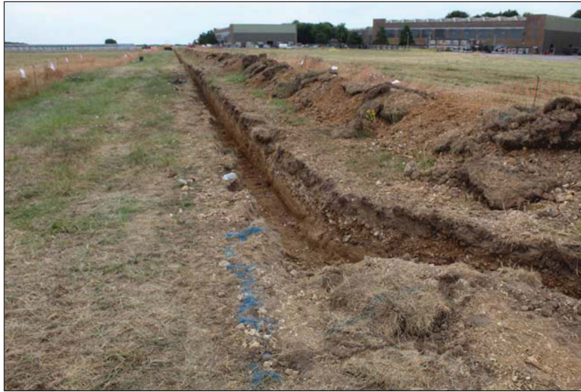
Plate 1. North route (Trench 2 turning into main Trench 1), looking South.
