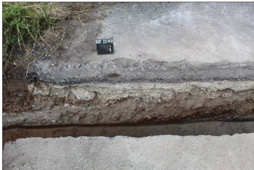
Plate 3. Trench section through road, looking South.
