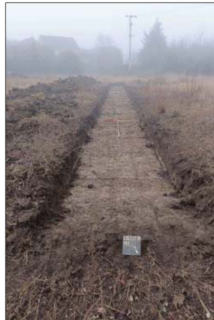
Plate 4. Trench 7, looking south-west, Scales: 2m, 1m and 0.2m.
