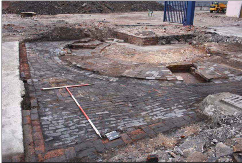
Plate 9. Wall 86 and blue brick working floor 85 around oven 1001, looking north-west, Scales: 2m and 1m.
