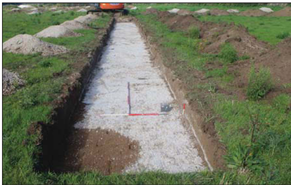
Plate 3. Trench 7, looking North-west. Scales: 2m, 1m and 0.20m.
