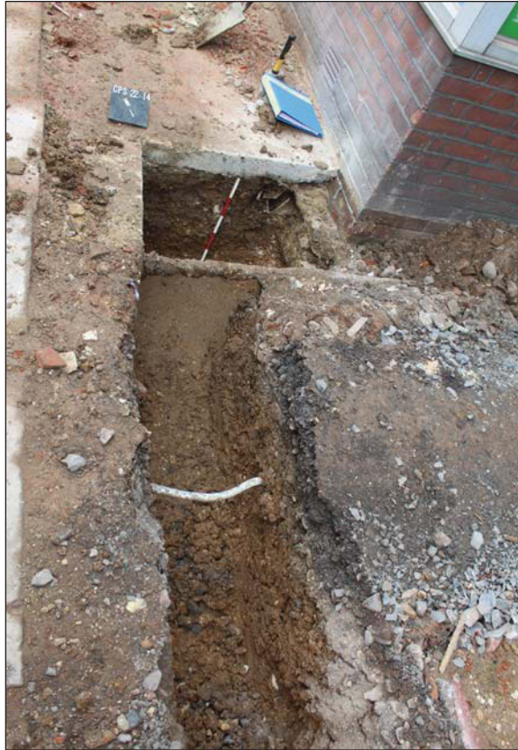
Plate 3. Trench, looking North East, Scale: 0.5m.
