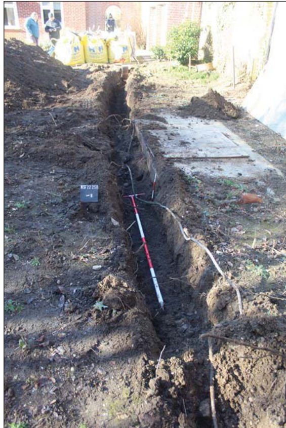
Plate 4. Drainage trench, looking North West, Scales: horizontal 2m, vertical 0.3m.
