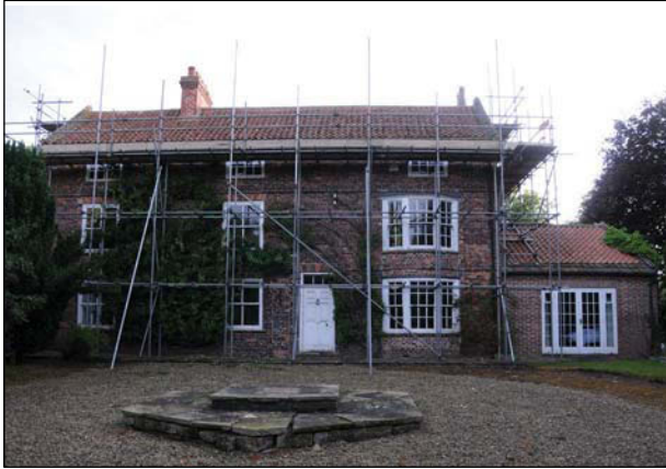
Plate 1. Exterior, house frontage, looking west.
