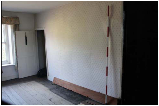
Plate 6. Looking SE, view of wallpapered wall and door to storage on the first floor, Scales: 2m.
