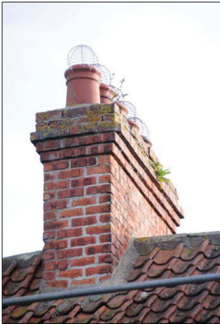
Plate 9. External chimney detail, looking west.
