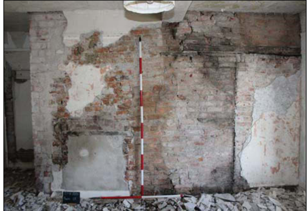
Plate 2. Looking north at the blocked up fireplace and opening on the first floor, Scales: 2m and 1m.
