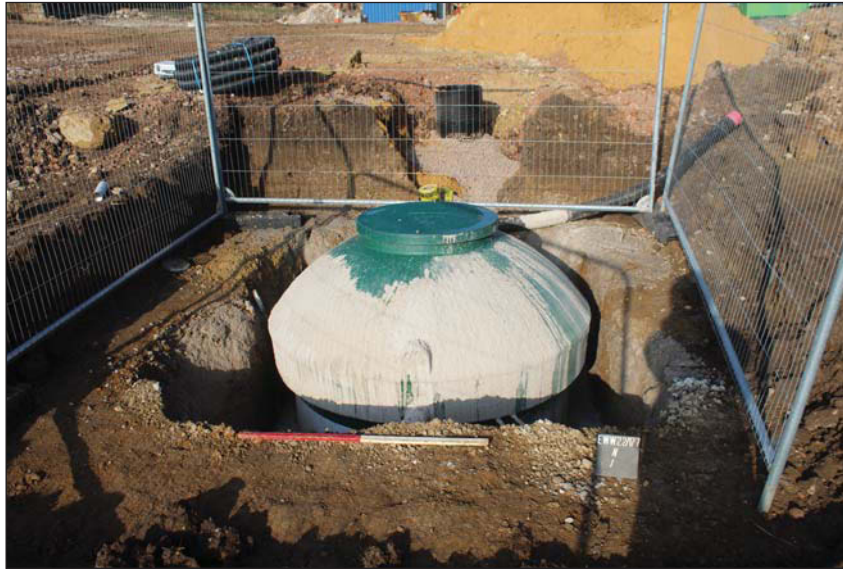
Plate 3. Excavated tank pit, looking North West, Scale: 1m.
