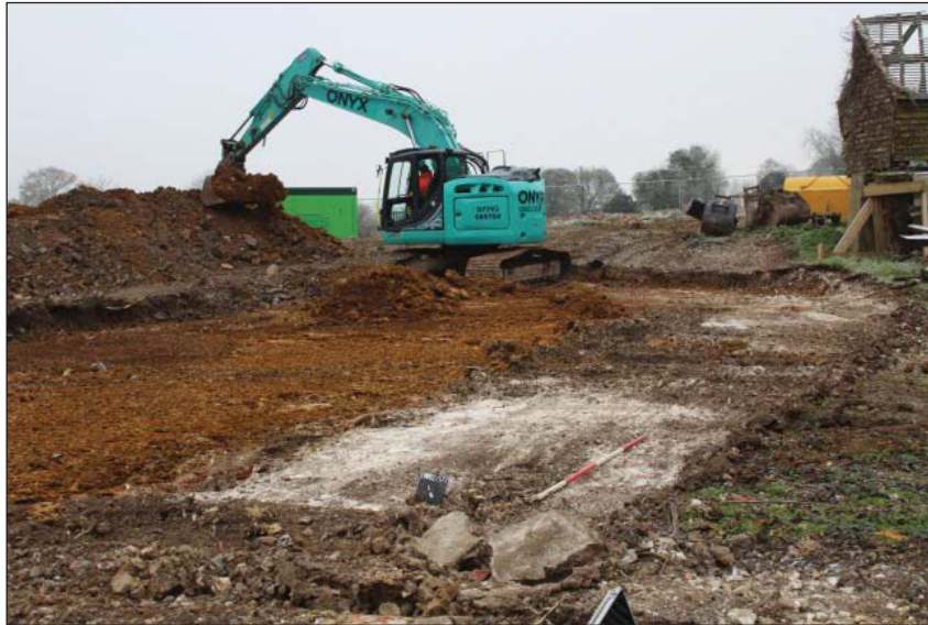
Plate 1. Ground reduction in progress, looking South, Scale: 2m.
