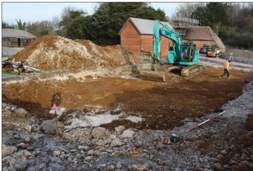
Plate 2. Stripped area, looking North, Scale: 2m.
