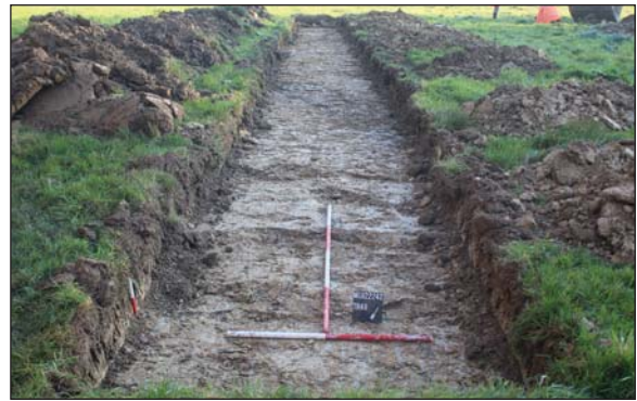
Plate 14. Trench 48, looking South-east. Scales: 2m, 1m and 0.2m.
