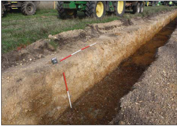
Plate 1. Pipe trench, looking east, Scales: 2m and 1m.
