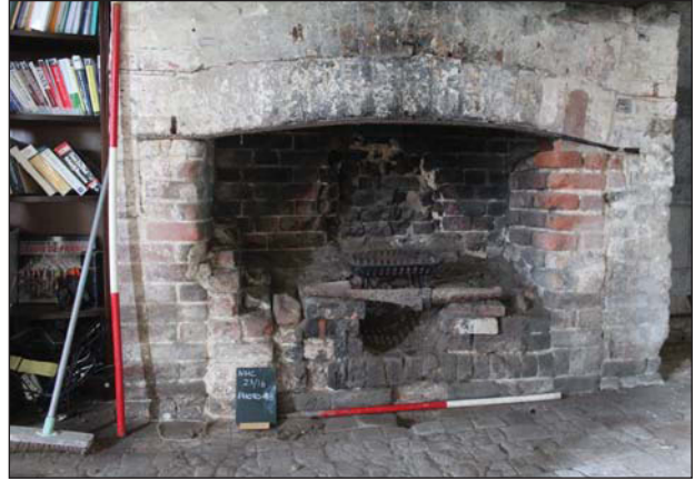
Plate 18. Main building 1: Fireplace detail looking East, Scales: 1x1m, 1x2m.
