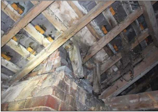
Plate 37. Main building 4:Chimney and roof detail, Looking North East
