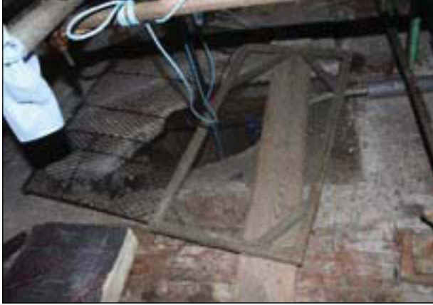
Plate 49. Well house: Well detail, looking north.
