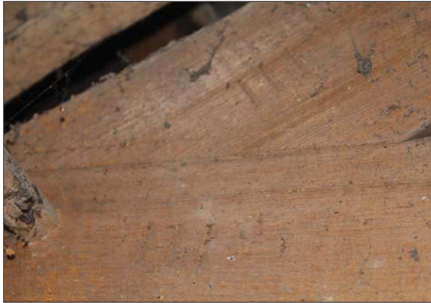
Plate 41. Main building 3: Carpenters marks 'III', looking South West
