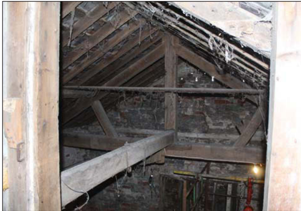
Plate 53. Well house: Truss detail, looking west
