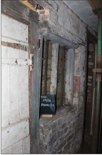
Plate 17. Main building 1: Oblique of window looking North East.
