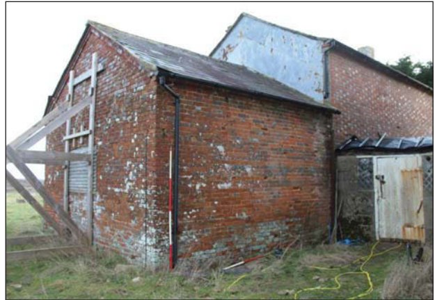
Plate 6. External: Oblique of well house looking North East. Scales: 1x1m, 1x2m.
