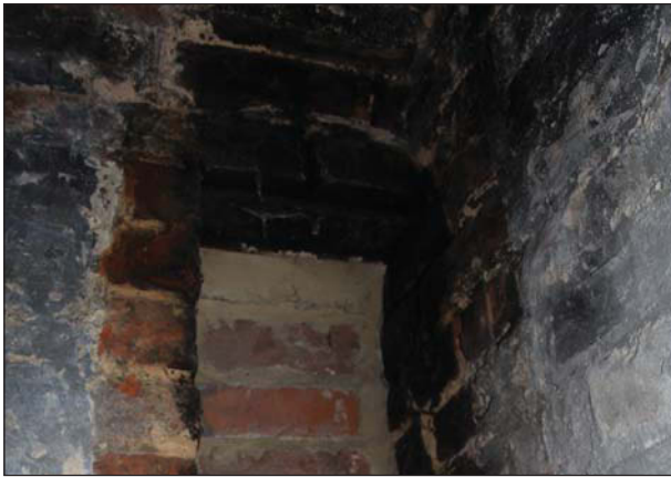
Plate 31. Main building 2: Alcove detail looking North West.
