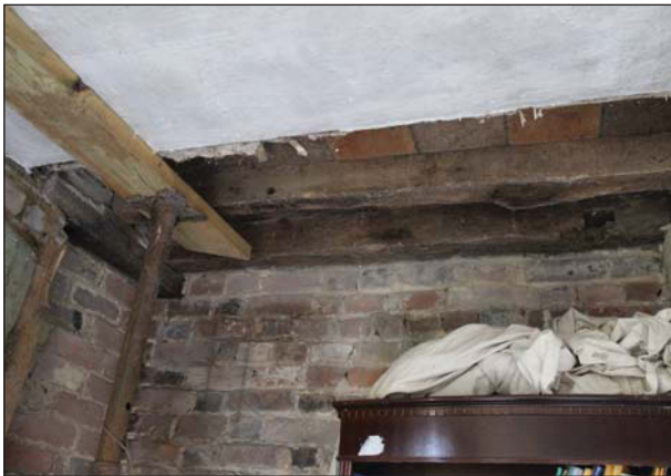
Plate 15. Main building 1, Ceiling detail looking East.
