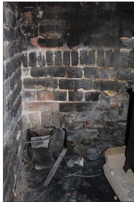
Plate 28. Main building 2: Bread oven detail, Looking North.
