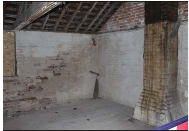
Plate 32. Main building 1: Oblique of room 3 to chimney stack, looking North East.
