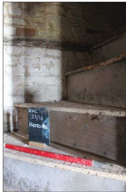
Plate 20. Main building 1: Main building 1, looking South, Scale:1m
