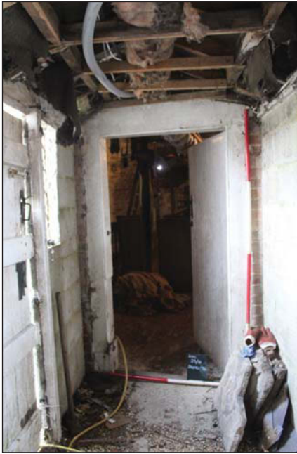
Plate 5. House link corridor: View to door looking North. Scales: 1x1m, 1x2m.
