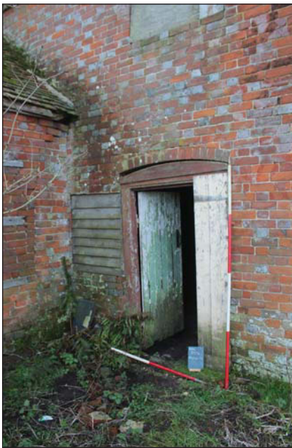
Plate 7. External: Door detail looking South West, Scales: 1x1m, 1x2m
