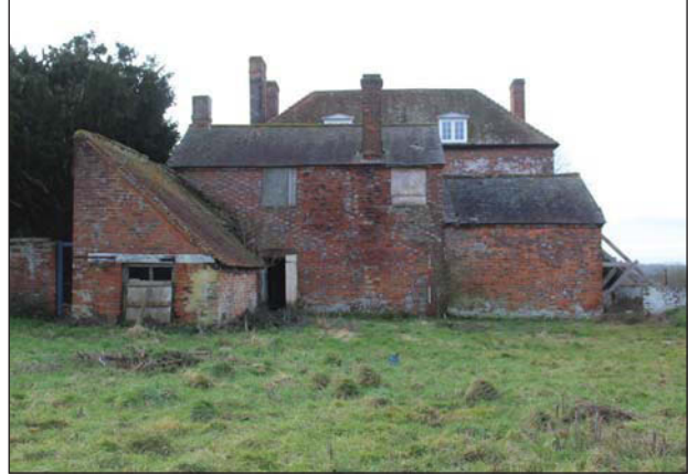
Plate 2. External: Rear of buildings with main house in the background, looking South, Scales: 1x1m, 1x2m.
