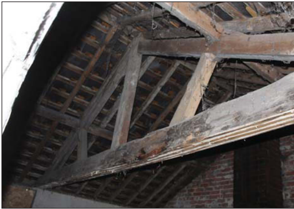
Plate 39. Main building : Gable end Looking East.
