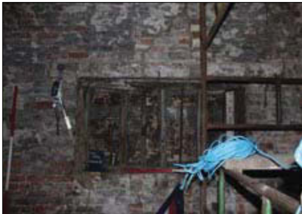
Plate 51. Well house: Window detail, looking west, 2m and 1m.
