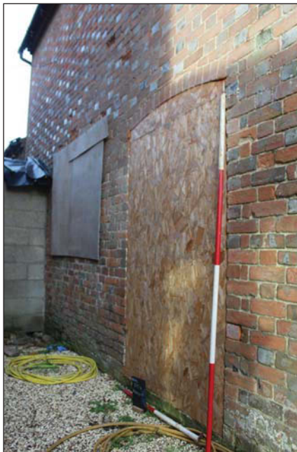
Plate 3. External: Door opening detail, looking North West, Scales: 1x1m, 1x2m.
