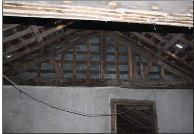
Plate 42. Main building 4, Gable truss detail looking North West
