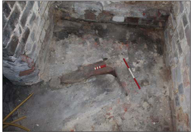
Plate 30. Main building 2, Floor detail looking North, Scales: 1x 0.1m, 1x0.3m
