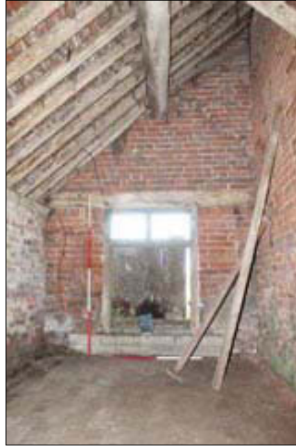
Plate 58. Rear building: North wall, looking north, Scales: 2m and 1m.
