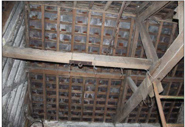
Plate 54. Well house: Roof detail, looking south
