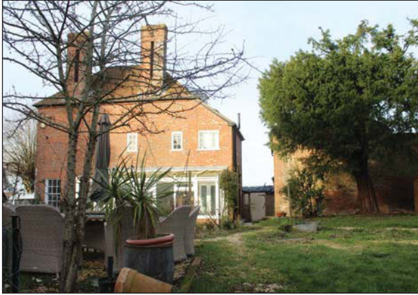
Plate 1. External: East elevation including the main house, looking South.
