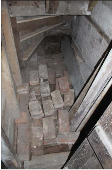
Plate 21. Main building 1: Under the stairs looking East
