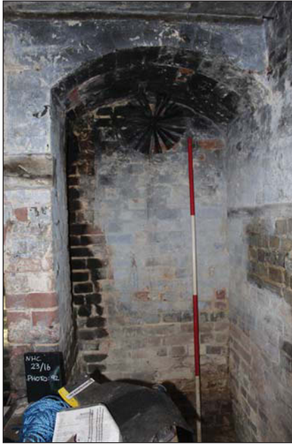
Plate 29. Main building 2: Alcove detail looking North, Scale: 2m
