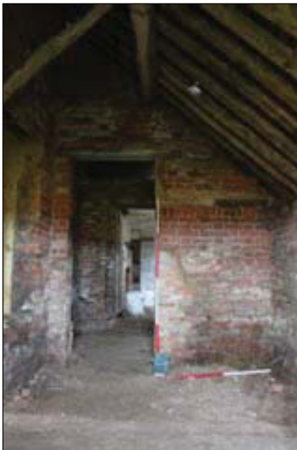
Plate 59. Rear building: South wall, looking south, Scales: 2m and 1m.
