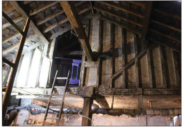
Plate 38. Main building 1, Floor detail looking West.
