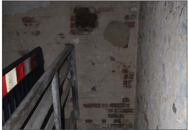
Plate 34. Main building 3, Down the stairs looking East.
