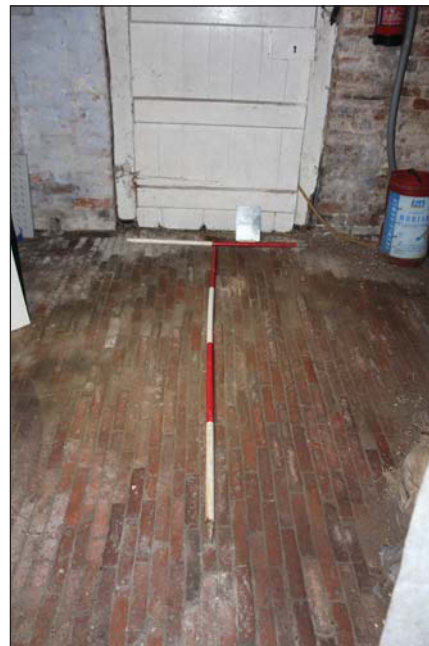
Plate 24. Main building 2: Floor detail looking South, Scales: 1x1m, 1x2m
