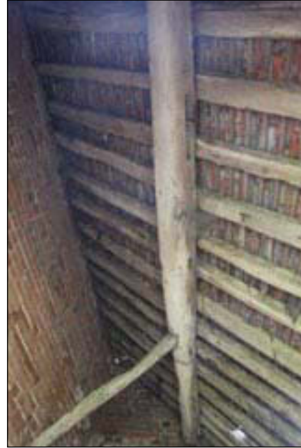
Plate 62. Rear building: Rood structure, looking south.
