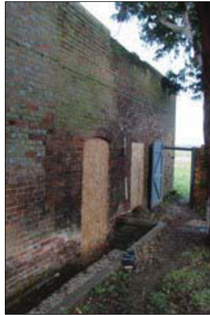
Plate 64. External: Oblique rear building and rear link, Scales: 2m and 1m.
