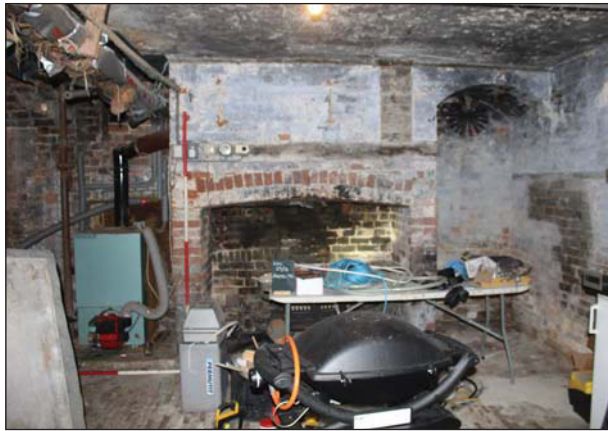
Plate 27. Main building 2: Chimney breast looking North, Scales: 1x1m, 1x2m
