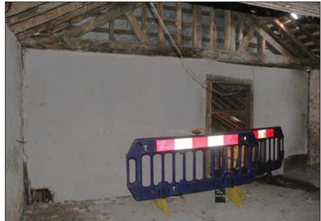
Plate 36. Main building 4: Oblique west wall looking West.
