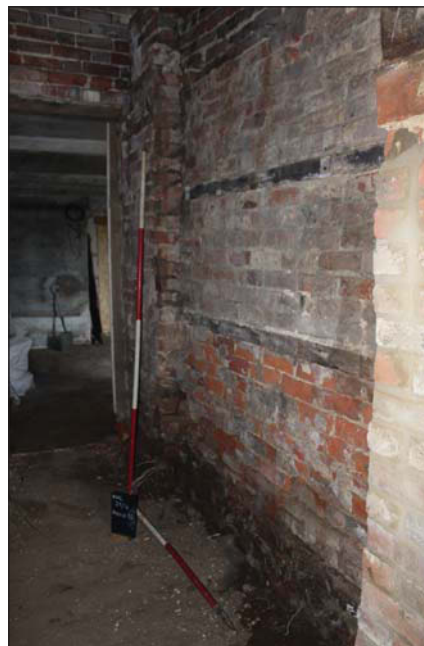
Plate 67. Rear link: Oblique west wall, looking south-west, Scales: 2m and 1m.
