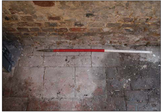
Plate 22. Main building 1, Floor detail looking West, Scale: 1m
