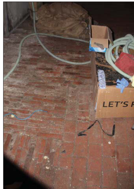
Plate 48. Well house: Floor detail, looking east
