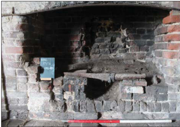
Plate 19. Main building 1: Fireplace detail, looking East, Scale: 1m
