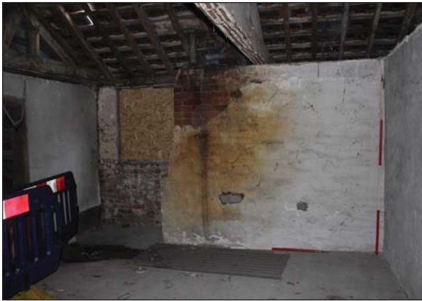
Plate 35. Main building 4: View to chimney breast looking North, Scales: 1x1m, 1x2m
