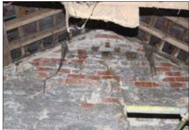
Plate 52. Well house: West gable end apex, looking west.
