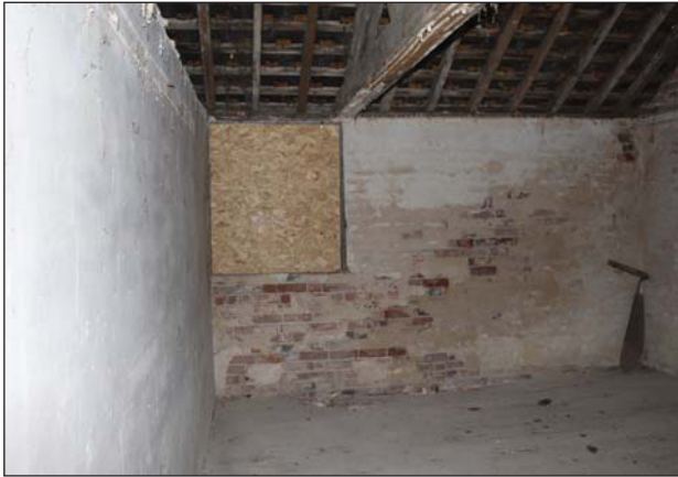
Plate 33. Main building 3: View to window looking North.
