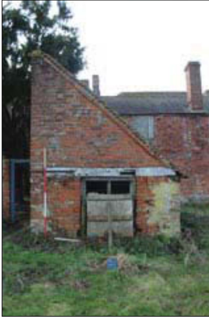
Plate 57. External: Rear building, north elevation, looking south, Scales: 2m and 1m.
