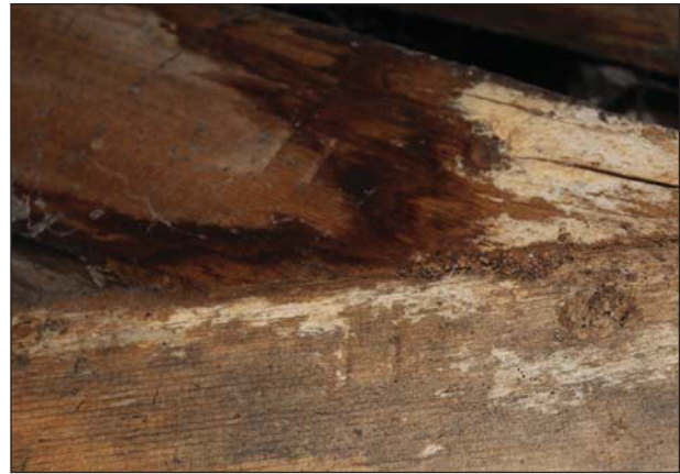
Plate 40. Main building 4: Carpenters marks 'II' looking North East.
