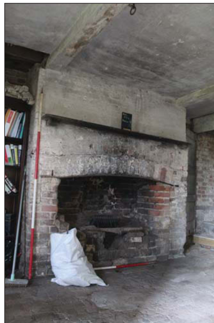
Plate 16. Main building 1, Fireplace, oblique looking South East, Scales: 1x1m, 1x2m
