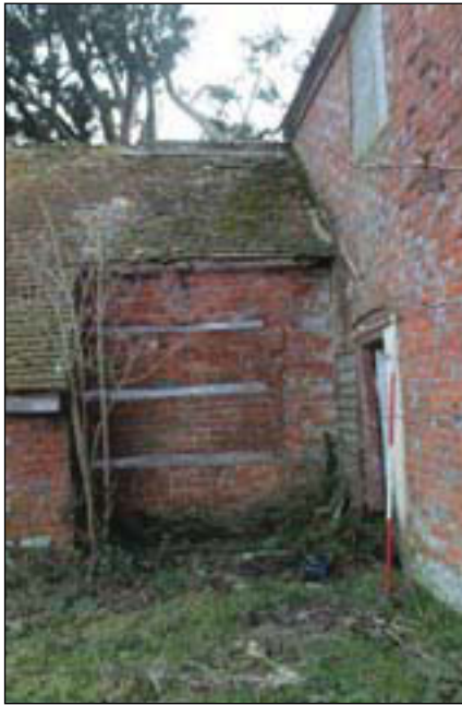
Plate 63. External: Rear link detail, looking east, Scales: 2m and 1m.
