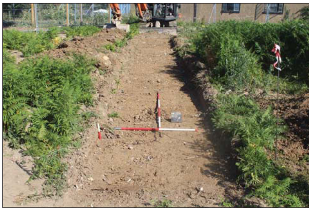
Plate 9. Trench 121, looking North West; Scales: 2m, 1m, 0.2m.
