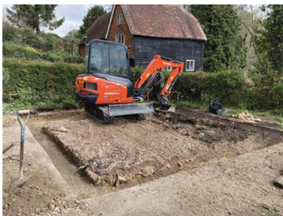
Plate 1. General view of site during ground reduction, looking north-east.
