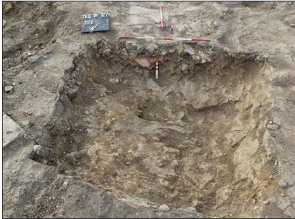
Plate 13 Foundation 322, looking south-east. Scales: 0.5m, 0.3m, 0.1m
