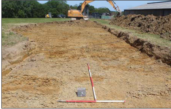
Plate 1. New Road Access. looking North East, Scales: 2m and 1m.
